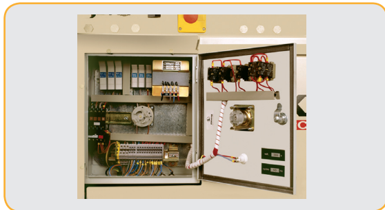
Electrical box with safety and integrated controls
